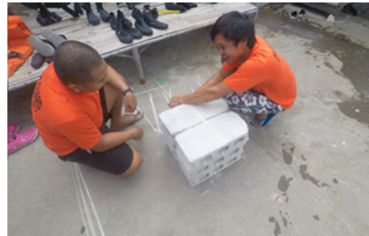
Lashing of the reef module on land shall be done with an assistant which will take about 20 minutes
